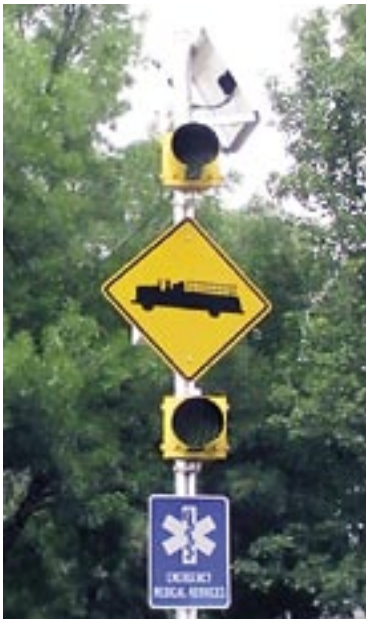
Typical Solar Powered EVCS
